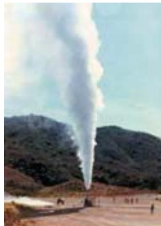
◀ **Fig. 2: Discharging well (LA-6) of the Aluto-Langano geothermal field. Total Depth = 2.5 km. Max. Temperature = 350°C.**
